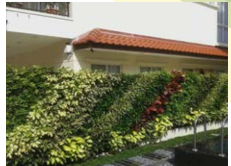
VERTICAL GREEN WALL
